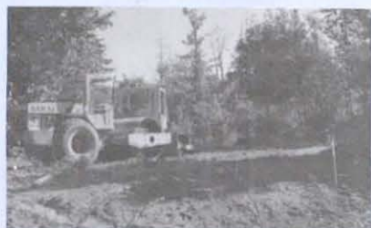
Work gets underway on Des Moines Creek Trail . . . . .page 2
